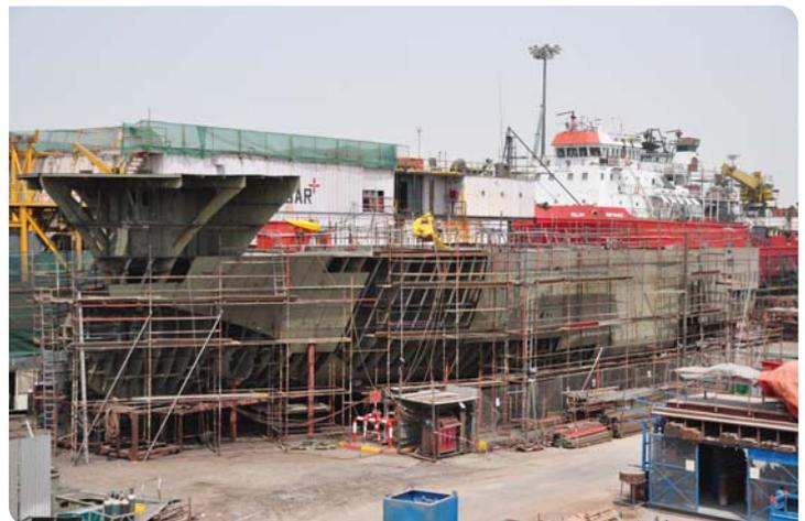
Hull construction of the DSV under progress
